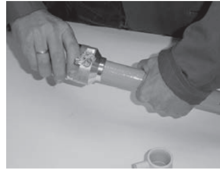
Fig. 3 On Bänninger Stabi-Pipes , the aluminum coating must be peeled off before jointing.
