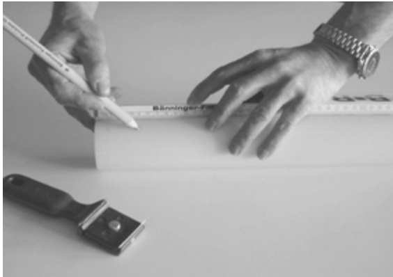
Mark the insertion depth of the sleeve
