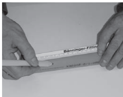
Fig. 5 Mark out the socket depth.
