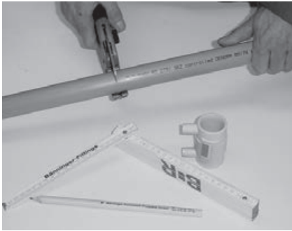
Fig. 1 Cut the pipe rectangularly with plastic scissors or with a pipe cutter.
