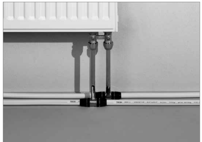
Radiator connection with radiator mounting tee
