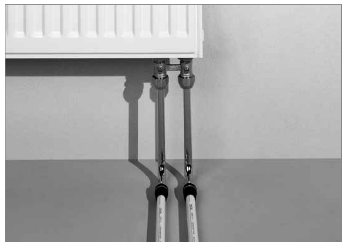
Radiator connection with radiator mounting elbow
