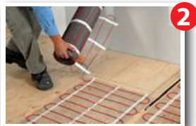
2 Cut the mesh to turn Never Cut the RED Cable
