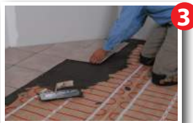
3 Install tile / floor coverings
