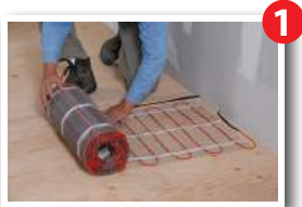
1 Unroll the self-adhesive mat onto the floor
