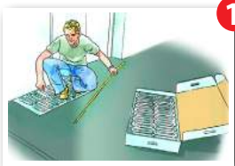
Lay out Reflect Plates
