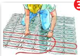
Install heating cable in grooves, pressing gently
